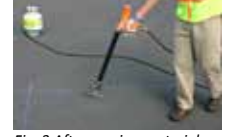
Fig. 3 After moving material aside, remove moisture from substrate
