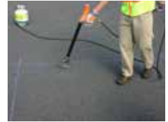
Fig. 1 Prepare area by removing debris with blower then remove moisture with heat torch
