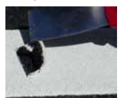
Fig. 4 Perform chisel test to verify bond. Evidence, as shown, of asphalt aggregate bonded to the underside of the lifted material indicates good adhesion.
